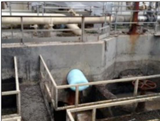
*CIPP liners typically cure overnight and the old sewer lines become structurally restored and can be put back into service within 24 hours.*
