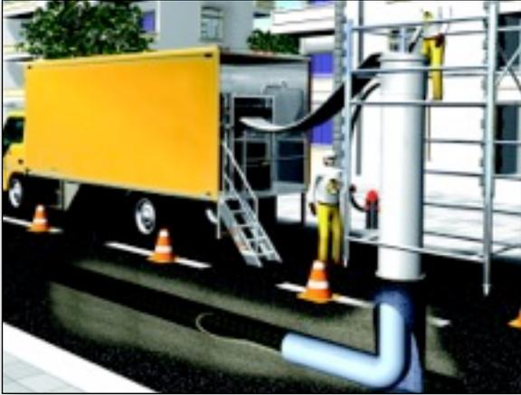
*A Typical set-up for CIPP pipe renewal. Small construction footprint and minimal surface disruption allow you to continue many of your daily operations above ground, while IPR relines your pipes below ground.*
